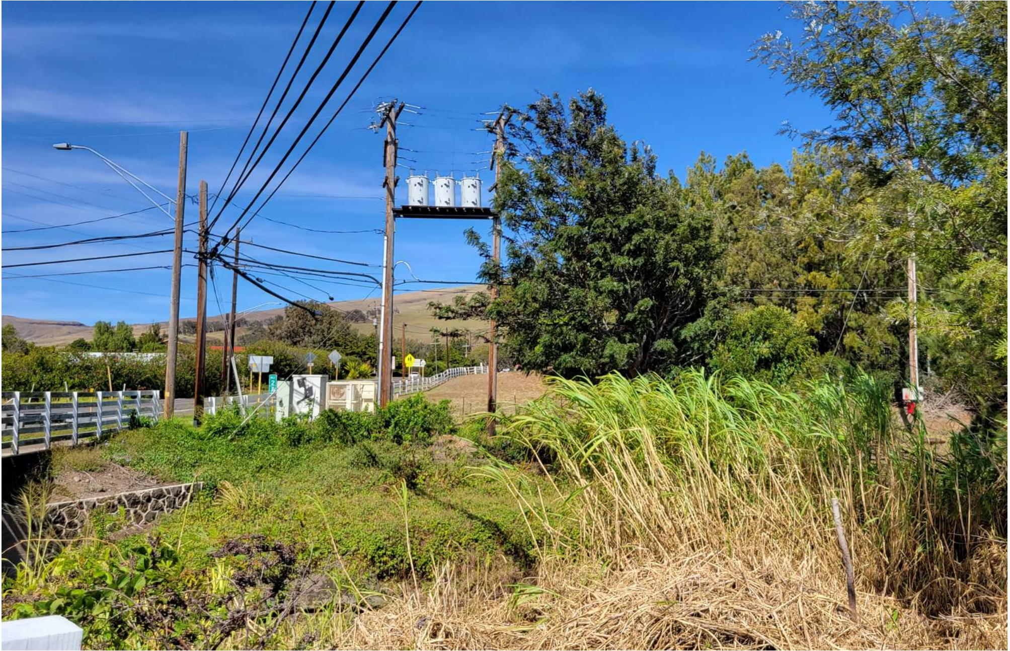
Photograph of Keanuiomano Stream with the existing Waiaka Bridge to the left
